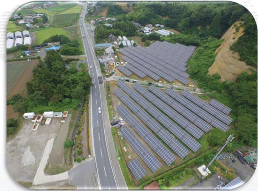
4MW Ground Mount, Japan
