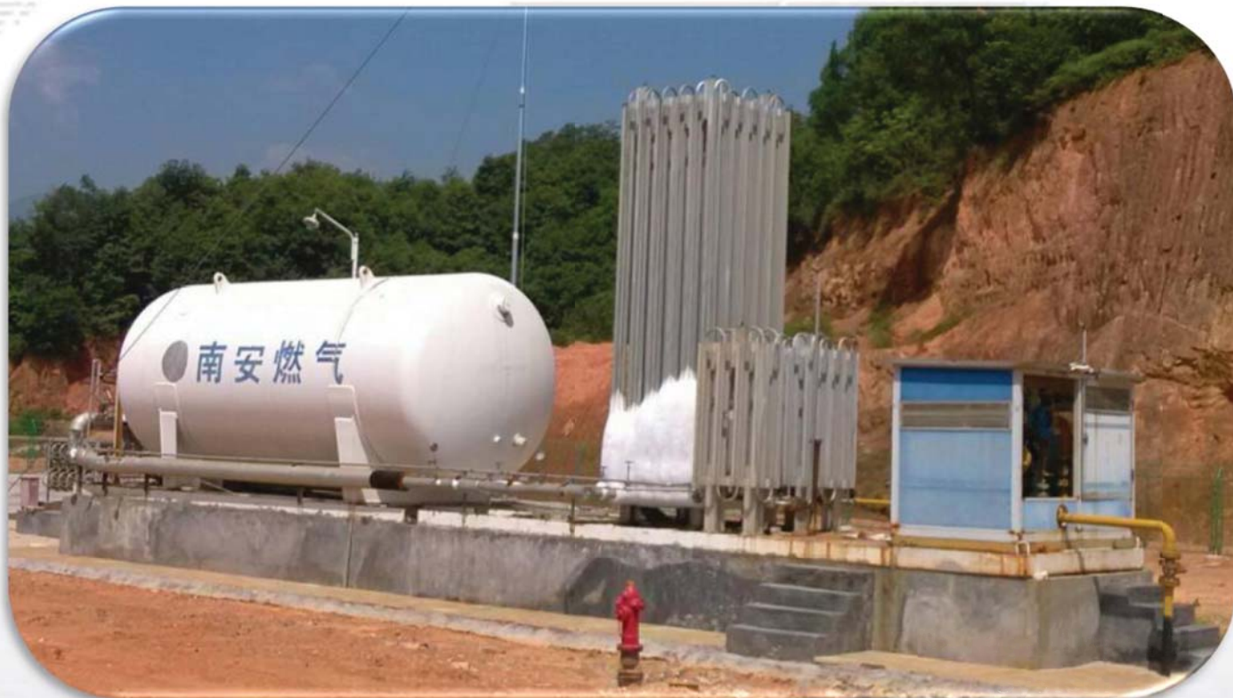
Natural gas station Daily supply capacity 30000m 3
