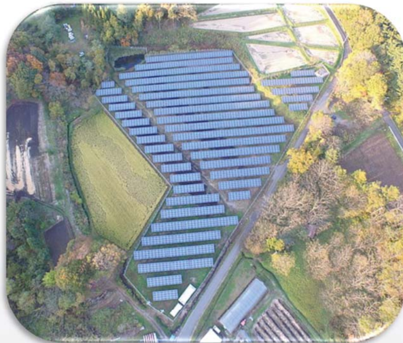
2.5MW Ground Mount, Japan
