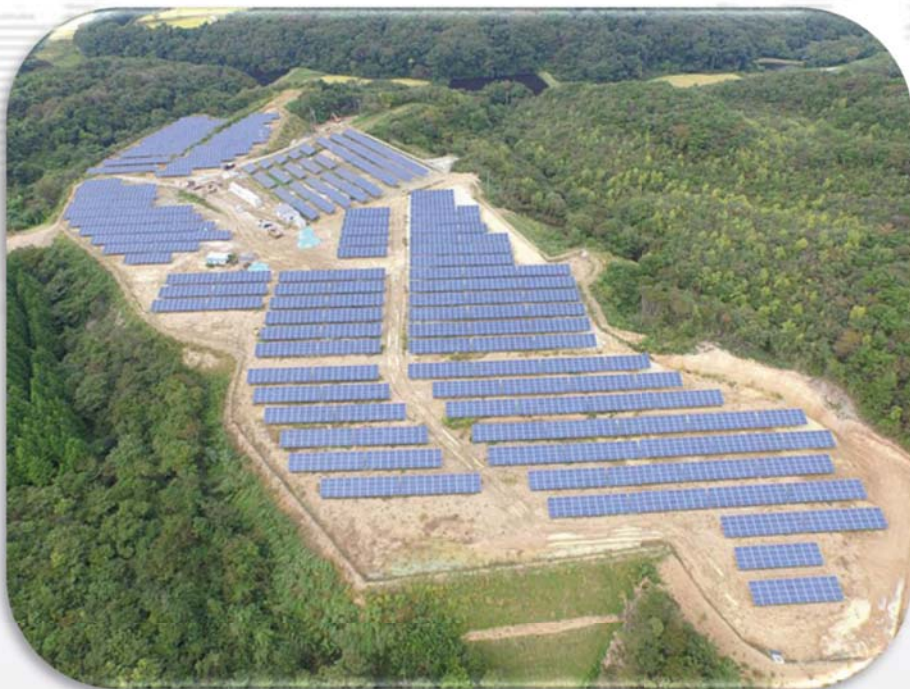
12MW Ground Mount, Japan
