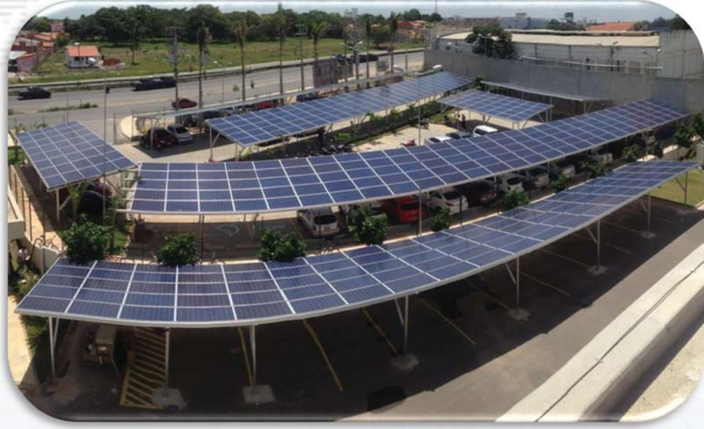
250KWSolar Carport, Brazil
