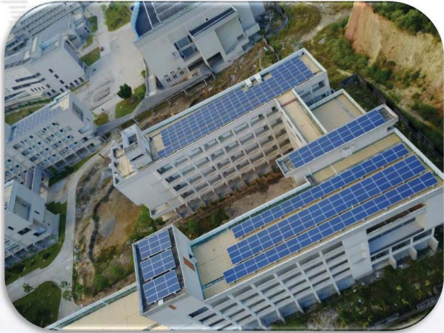
350KW School Flat Roof, Nan'an, Fujian
