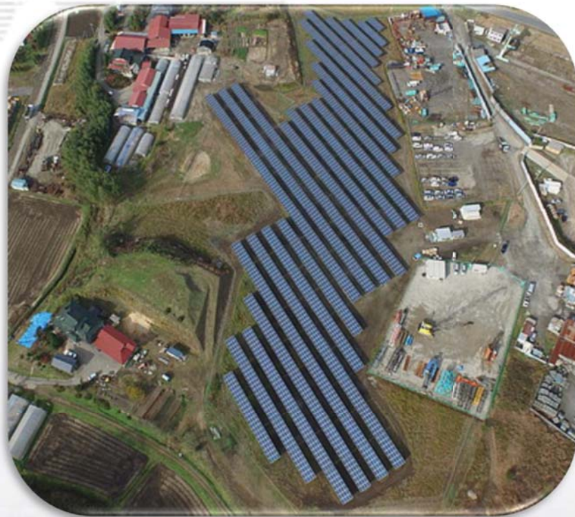
1.5MW Ground Mount, Japan
