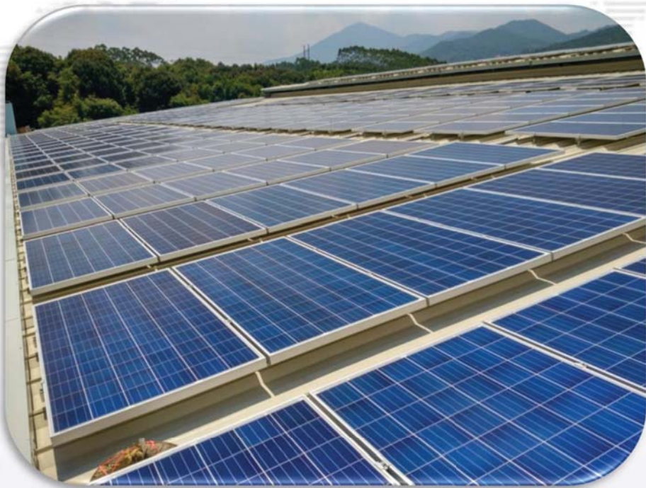
350KW Factory Metal Roof, Nan'an, Fujian
