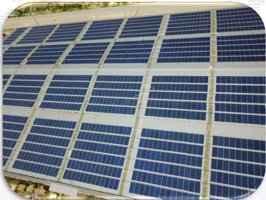
810KW Factory Metal Roof, Tong'an, Fujian
