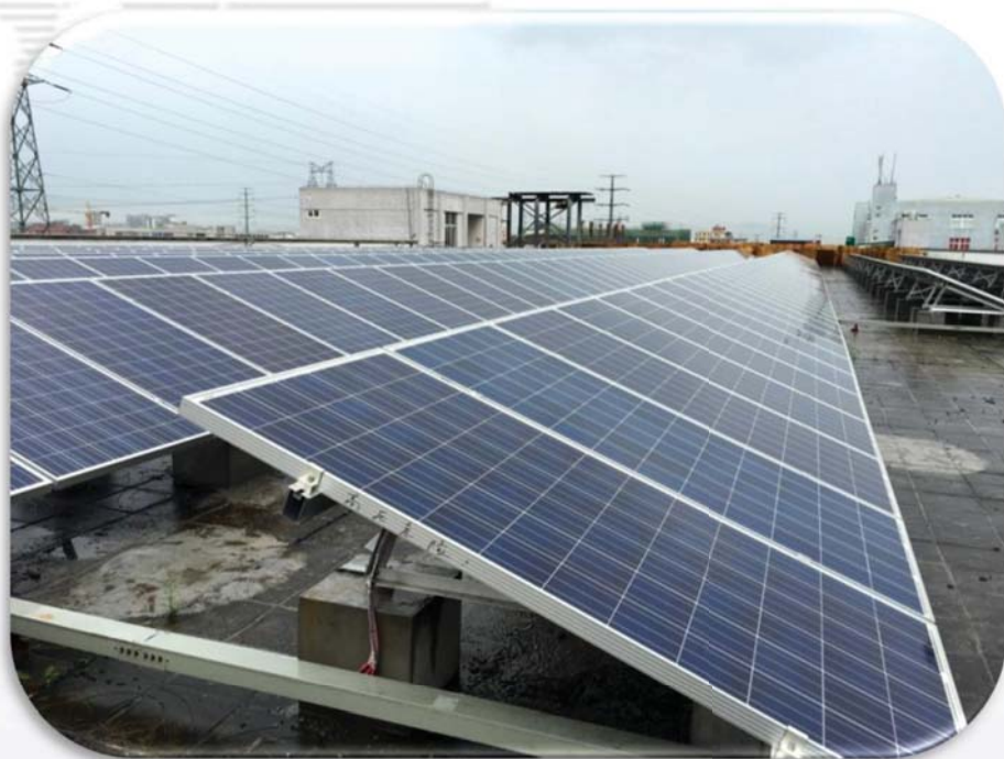
250KW Office Concrete Roof, Tong'an
